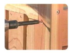
Once again they drilled clearance holes with a countersink bit so that the rust resistant screws were flush with the wood.
