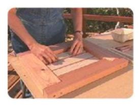
Once the frames for the end pieces were complete, they filled in the centers with wooden slats, which they laid in place temporarily.
