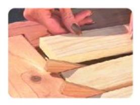
Next she turned the frame over, applied some glue to the ends of each slat and laid them on top of the keeper.
